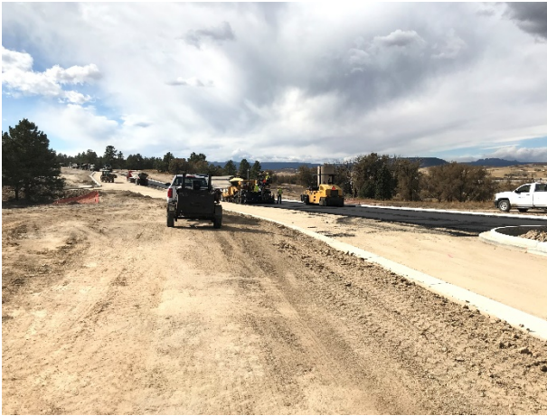
Montaine Cir Grading
