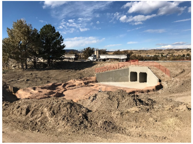
Box Culvert into Pond A
