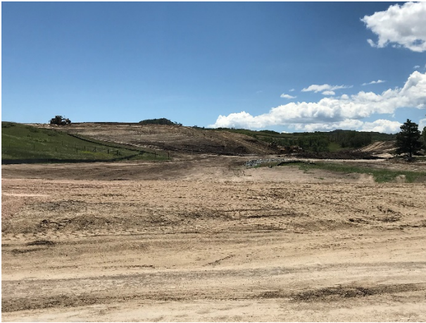
Montaine Cir Earthwork
