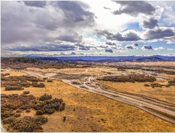
Montaine Cir Earthwork
