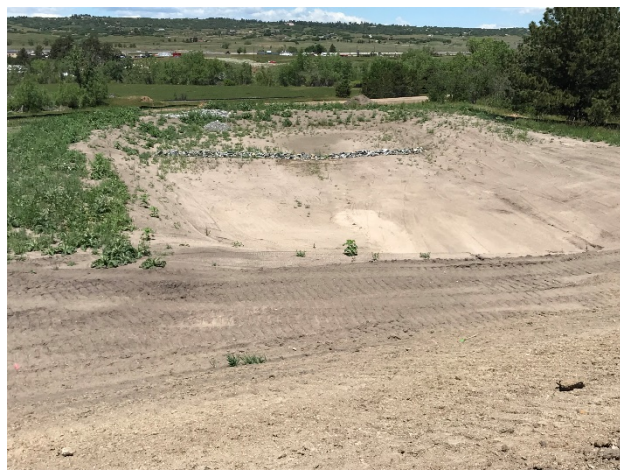
Montaine Cir Sediment Basin
