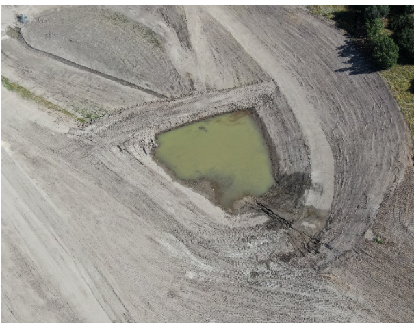
Montaine Cir Sediment Basin Aerial
