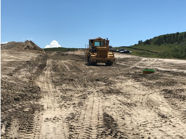
Montaine Cir Earthwork
