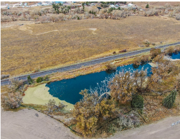
Aerial of Stormwater Easement
