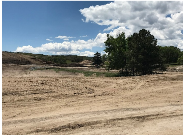
Montaine Cir Earthwork
