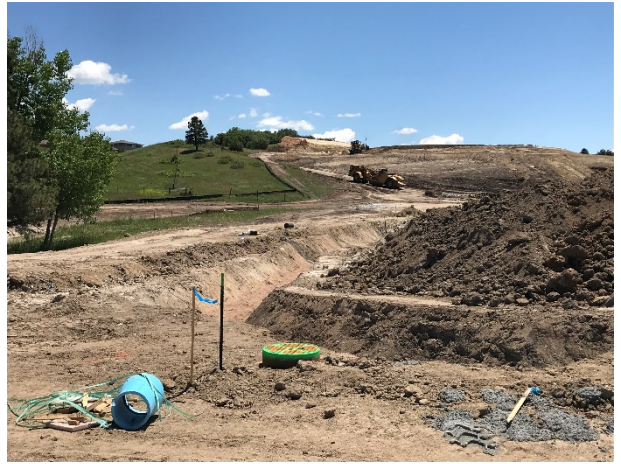
Montaine Cir Water and Sewer Mains
