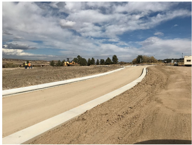
Road Base – Montaine Circle Earthwork
