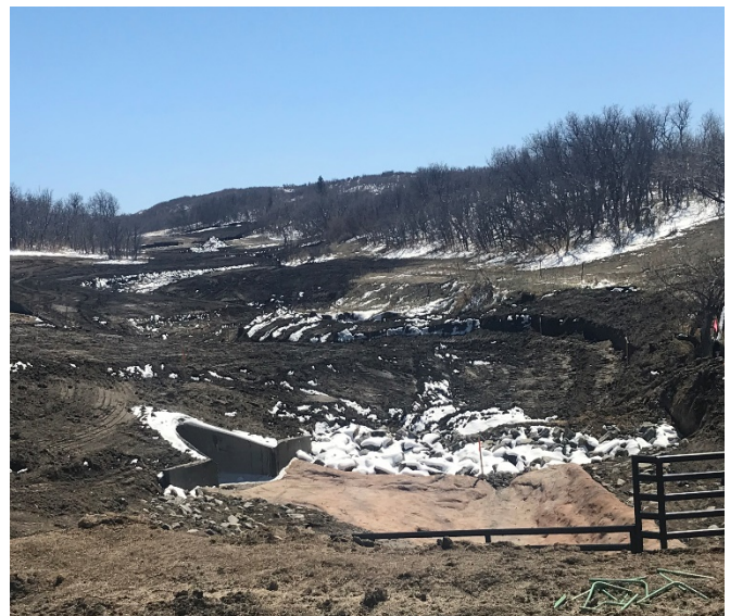
Filing 3 Storm Sewer – Montaine Cir Crossing
