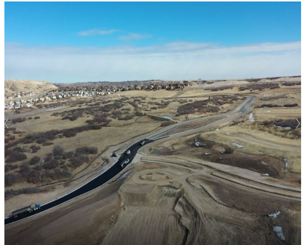
Montaine Cir & Filing 3 Earthwork
