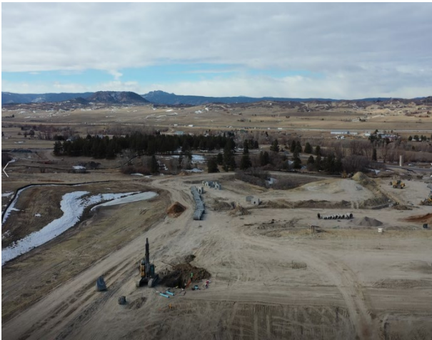
Filing 2 Earthwork & Utilities
