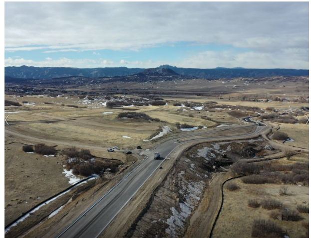
Montaine Cir and Filing 3 Earthwork
