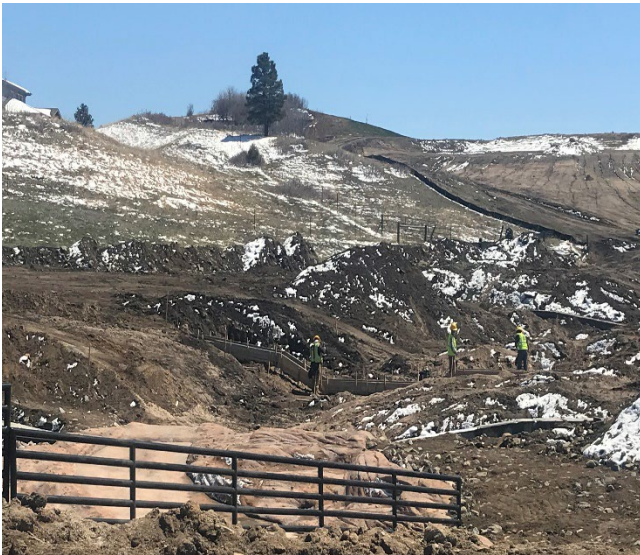
Filing 2 Storm Sewer – Montaine Cir Crossing
