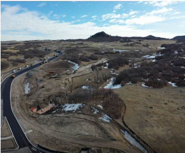
Montaine Cir & Filing 3 Earthwork
