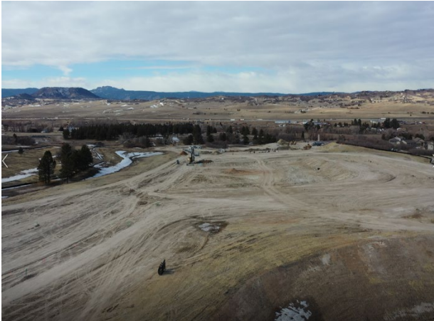
Filing 2 Earthwork & Utilities
