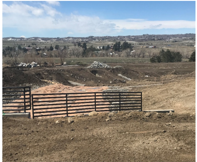
Filing 2 Storm Sewer - Montaine Cir Crossing
